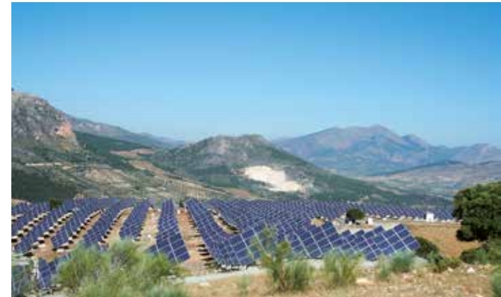
KPV ground mounted PV park / Spain
